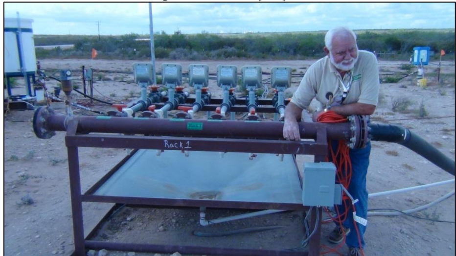
Image 3: Production pump rack with individual well monitors
