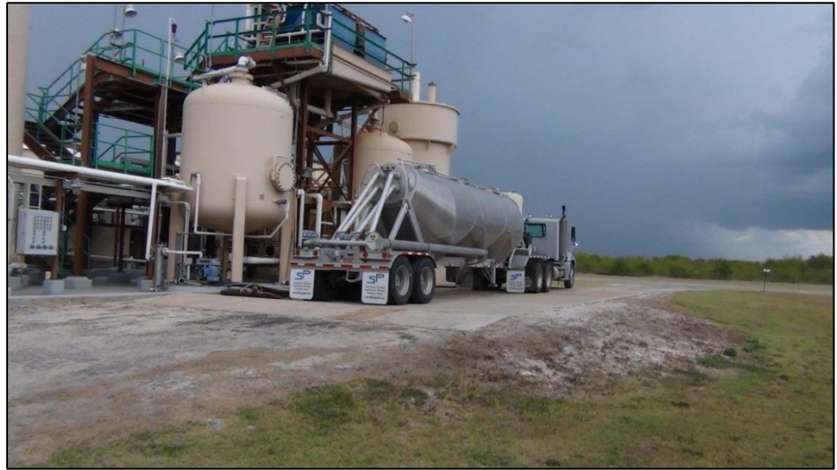
Image 4: Truck with resin tank at Hobson
