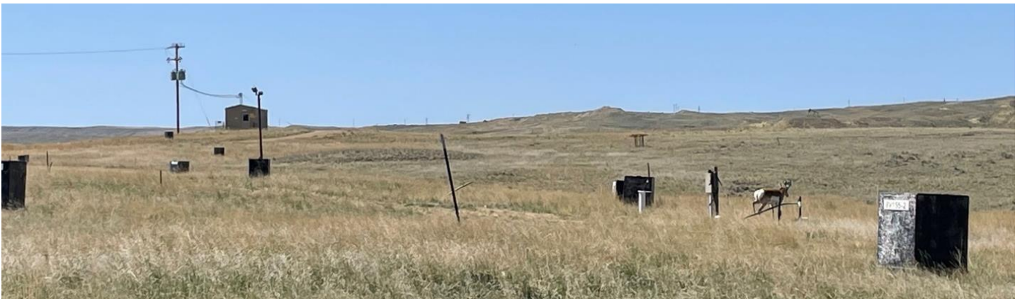
Figure 8: Christensen Ranch – Unit 8 wellfield
