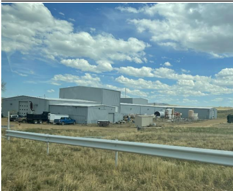
Figure 2: Irigaray Central Processing Plant
