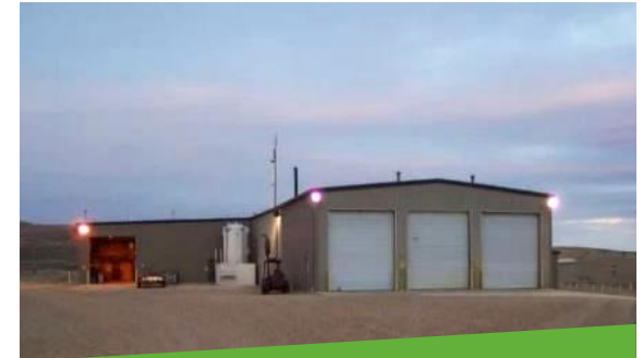
Christensen Satellite Plant
