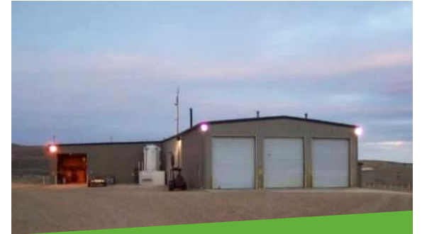
Christensen Satellite Plant
