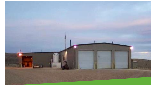
Christensen Satellite Plant
