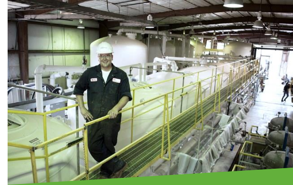
Christensen Satellite Plant
