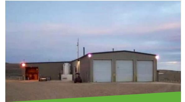
Christensen Satellite Plant
