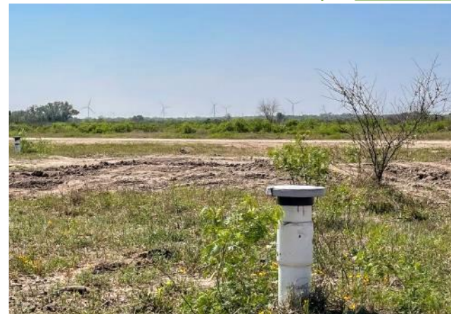
Cased monitor wells in the Production Area 1, at Burke Hollow Project
