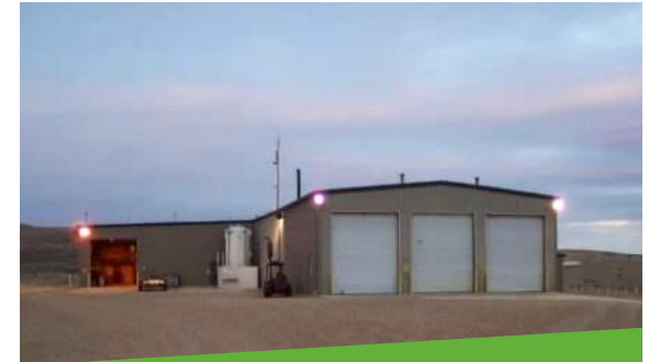
Christensen Satellite Plant
