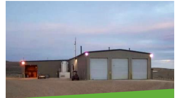
Christensen Satellite Plant
