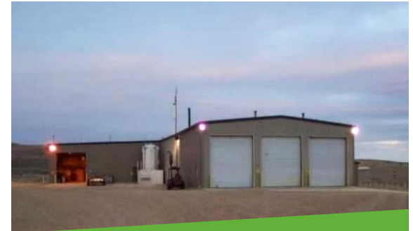
Christensen Satellite Plant
