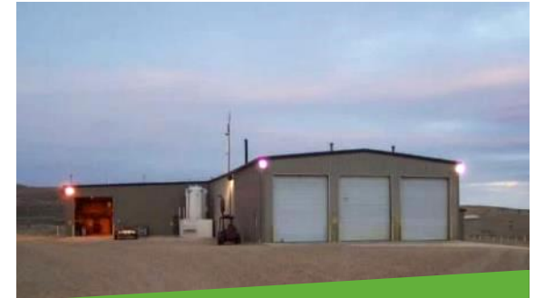
Christensen Satellite Plant
