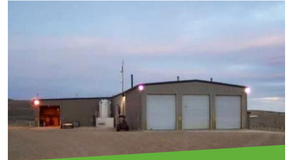
Christensen Satellite Plant
