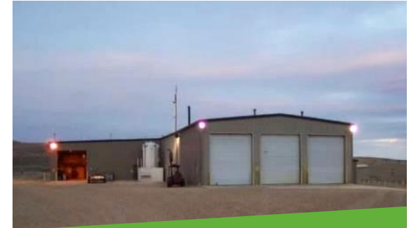
Christensen Satellite Plant
