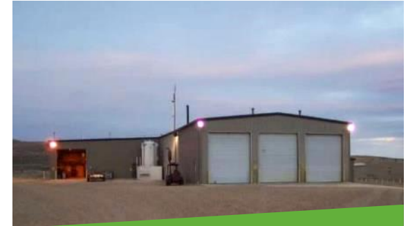
Christensen Satellite Plant
