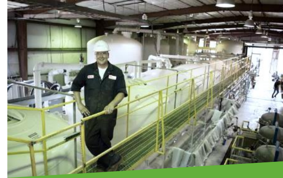
Christensen Satellite Plant
