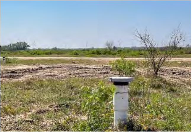
Cased monitor wells in the Production Area 1, at Burke Hollow Project
