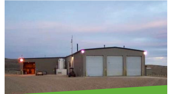
Christensen Satellite Plant
