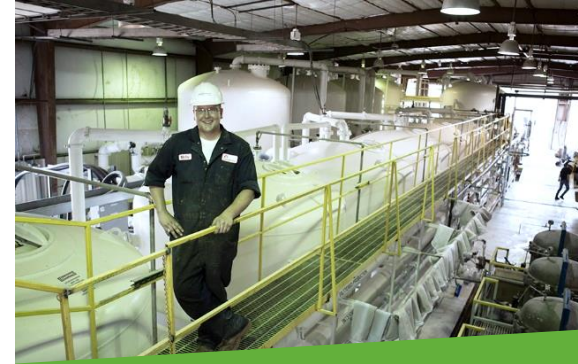
Christensen Satellite Plant
