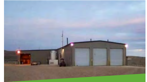
Christensen Satellite Plant
