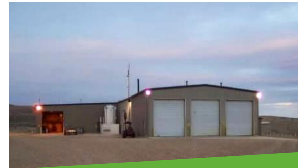
Christensen Satellite Plant
