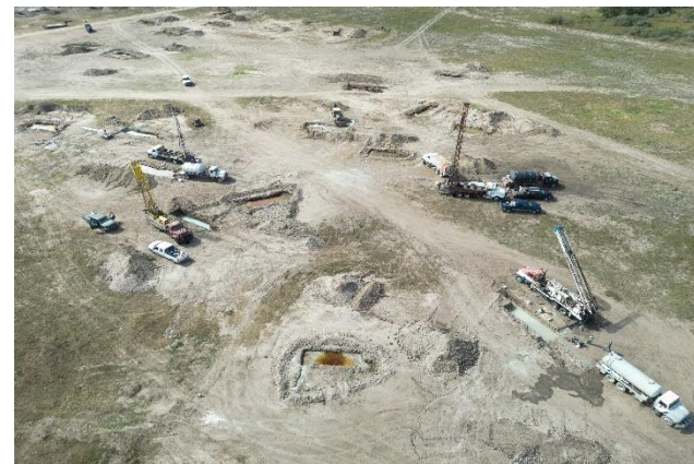
Drilling, Burke Hollow
